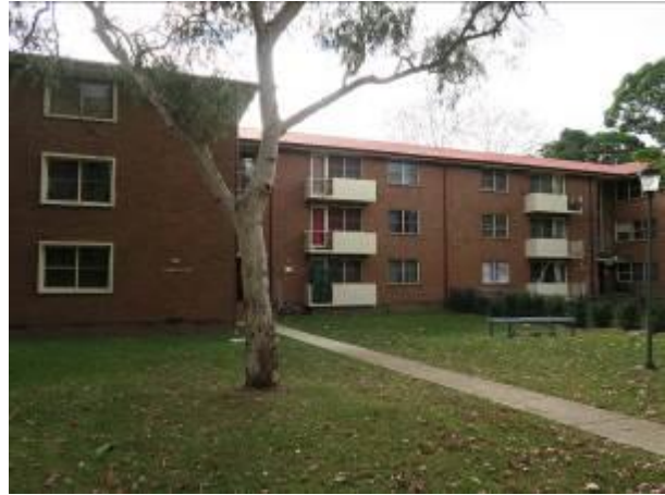
Picture 4 – Ground surface visibility and exposure within the yard areas of residential buildings
